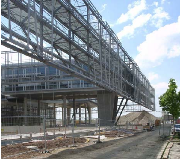
Spatial steel construction - reality
